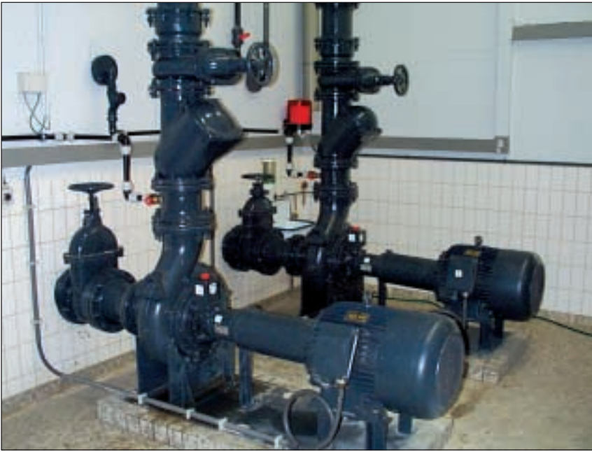
Robot dry installed pumps, the ultimate solution for solids handling applications. Above two BT6050 pumps managing the sewage system at Amsterdam airport "Schiphol".
