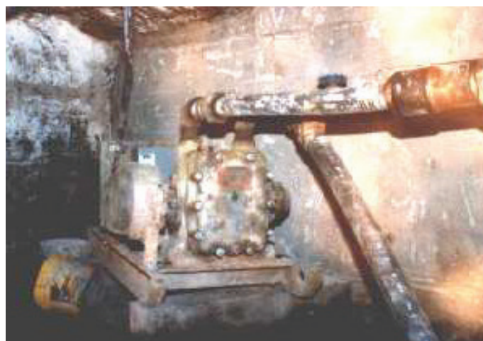
▲ Rugged conditions underground mining duties
