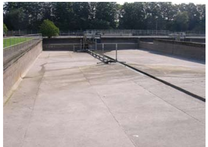
Large installation in UK: 48m x 21m tank with single 37 kw pump with manifold as an alternative to a multi pump solution
