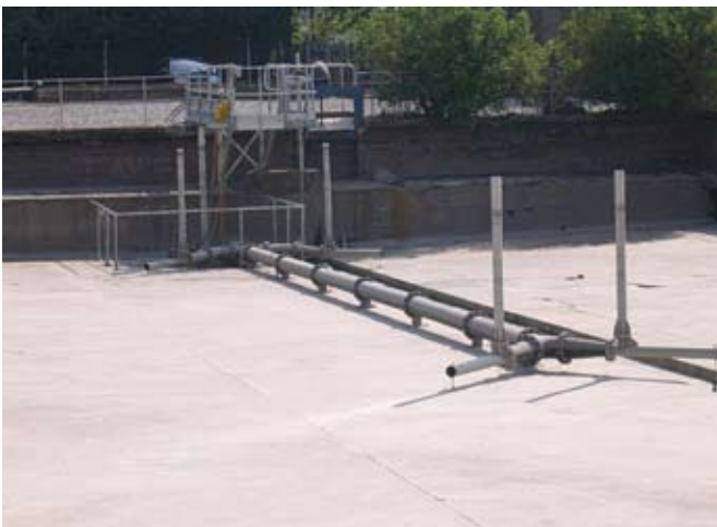
Large installation in UK: 48m x 21m tank with single 37 kw pump with manifold as an alternative to a multi pump solution
