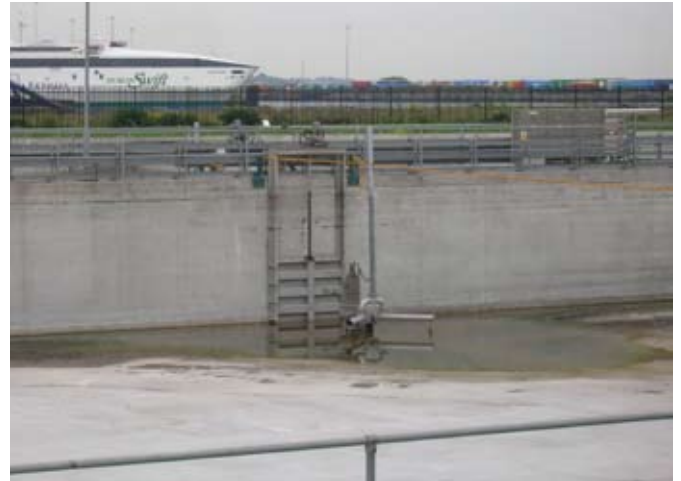
Large installation in Ireland: 6 tanks – average dimension 37m x 89m with 36 x 18.5 kw pumps used with twin barrels
