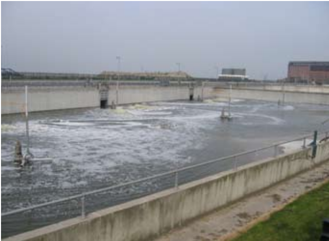
Large installation in Ireland: 6 tanks – average dimension 37m x 89m with 36 x 18.5 kw pumps used with twin barrels
