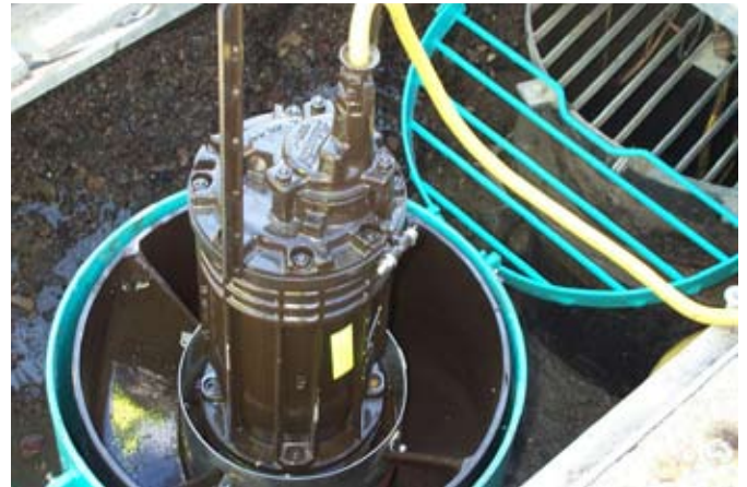
Pump being lowered into tube
