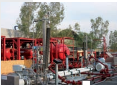
Well testing disposal, Abu Dhabi, UAE
