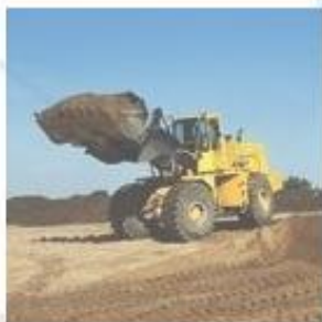
Construction site dewatering
