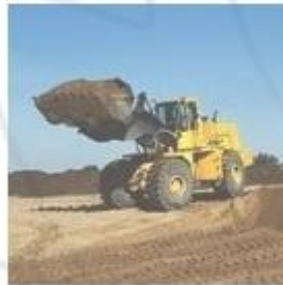
Construction site dewatering
