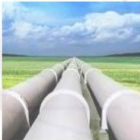
Municipal water supply
